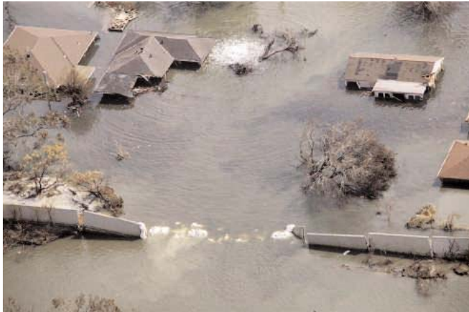
A broken levee on the east side of the London Avenue Canal in the Gentilly neighborhood of New Orleans, 11 September 2005.
